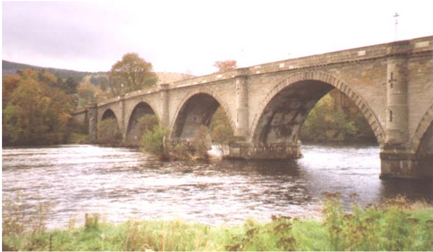
Telford's 1809 bridge at Dunkeld which must have been a familiar sight to the Frasers.
