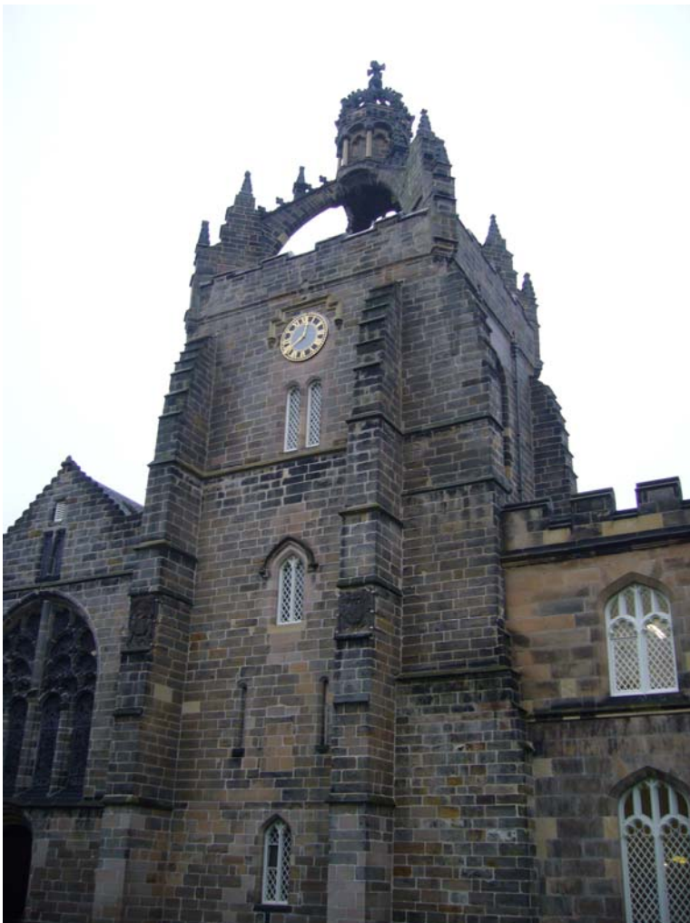
The Chapel tower
